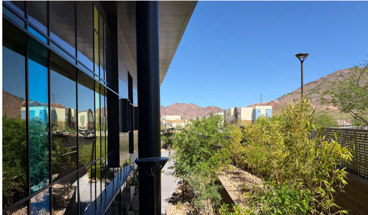
The windows of this Nevada State University building allow natural light throughout the interior spaces, while the deep roof overhangs help protect building occupants from the intensity and heat of direct sunlight.
