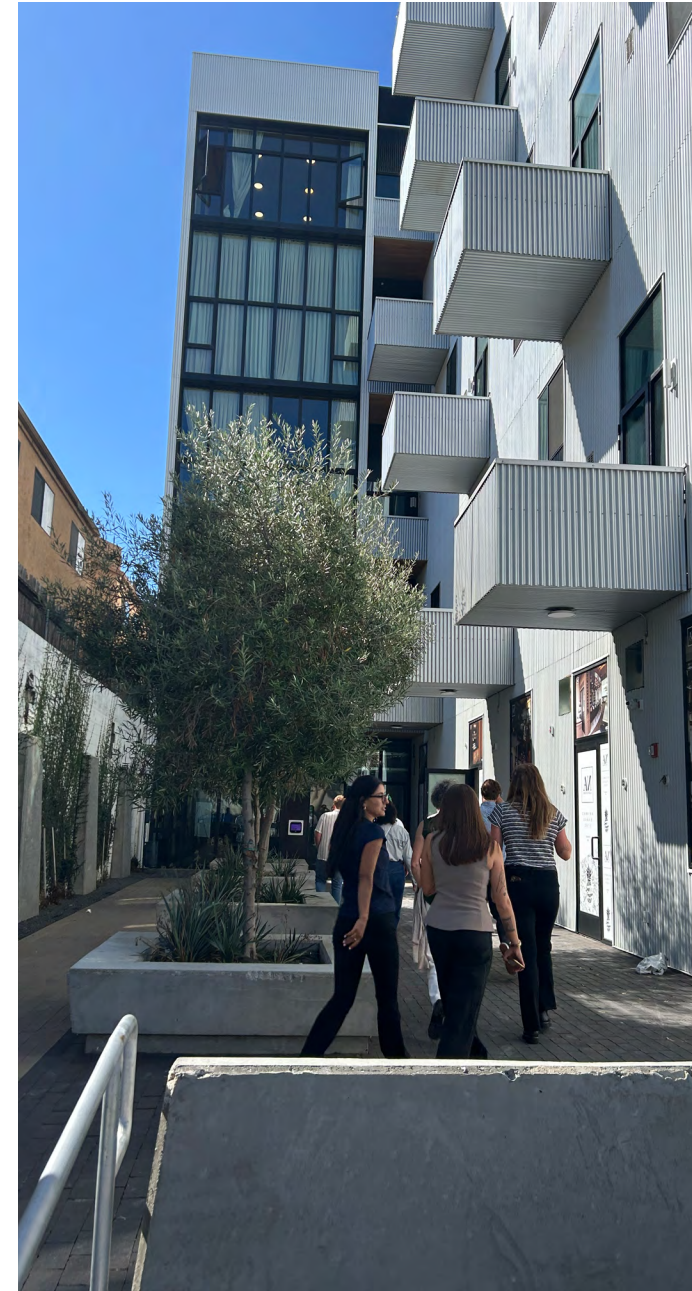
This building features a combination of mass timber construction for the structure and recycled material for the cladding around the units' balconies.
